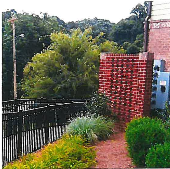
Figure 6-7-5 Service area screening
