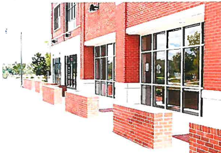
Figure 6-6-6: Facade transparency (windows) along a street facade
