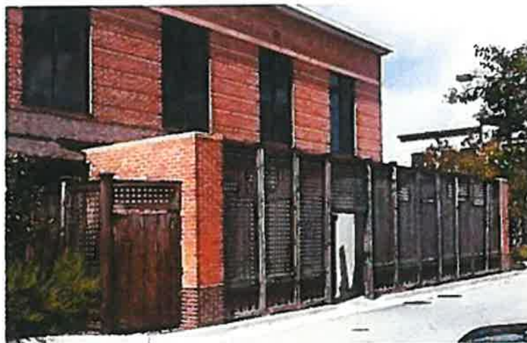
Figure 6-5-9: Screening elements integrated with the building
